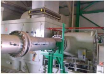
**Sontrach's SC3** gas compression station is equipped with the Solar Titan 130 gas turbine and auxiliary equipment shown here. The turbine generates roughly 20,000 hp, helping transport gas from Algeria's Hassi R'Mel field to Europe (Fig. 2).
