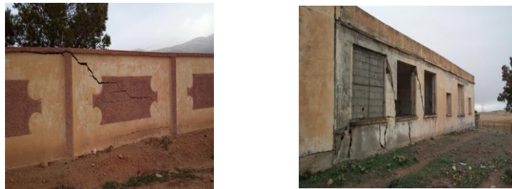
Fig. 3. Field photographs showing the shrinking-swelling soil problems in the study area.
