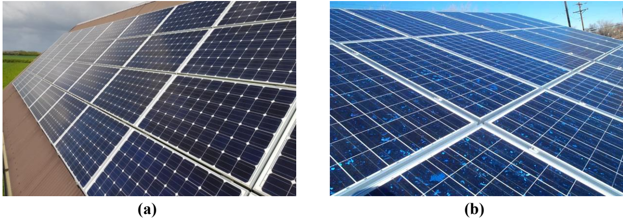
Figure I.4: Silicon crystalline PV module: monocrystalline (a), polycrystalline (b)
