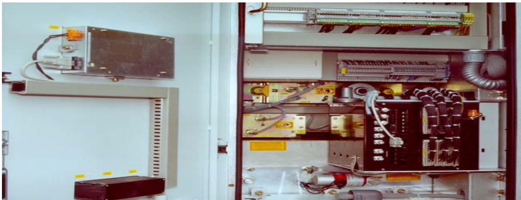
Figure 3.7 Mounting of the Central Unit in the LV compartment and the HMI on the door
